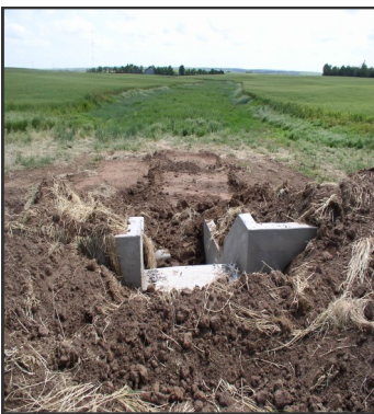
Concrete block structure installed to correct erosion issue
