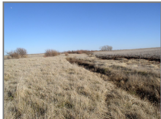
Left side of waterway is high due to sedimentation. Cuts to the right are a result of water needing a place to go.
